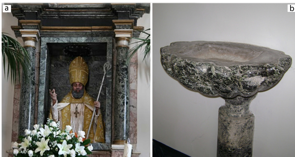
Fig. 1 - Examples of use of serpentinite rocks for artefact. a) pillars in altar; b) baptismal font.
