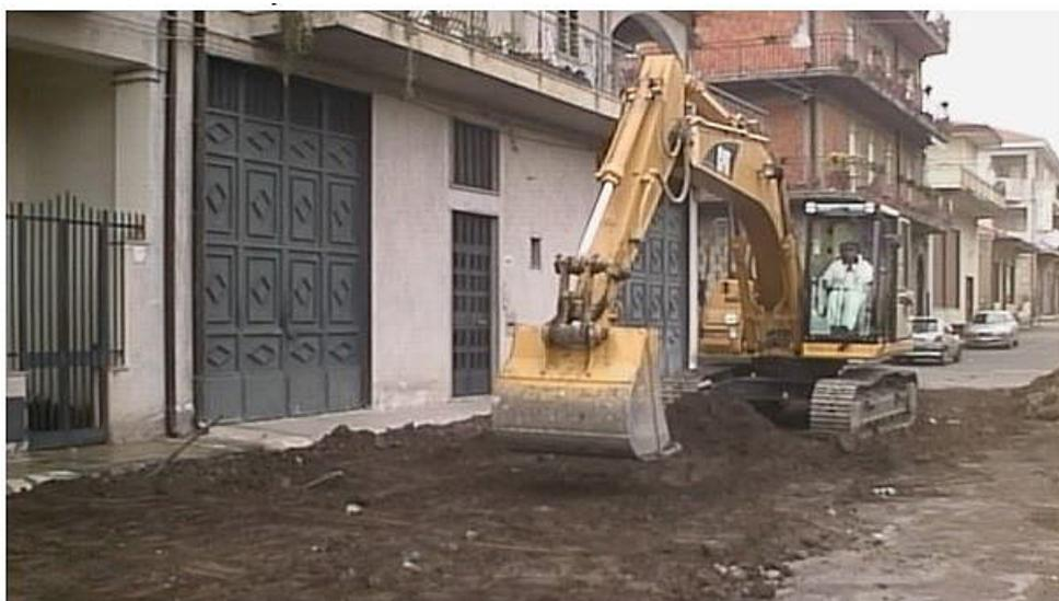
Fig. 3 - Work on removing the old paving in Biancavilla.
