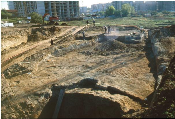
Fig. 1 - View of the excavation site - November 1981.
