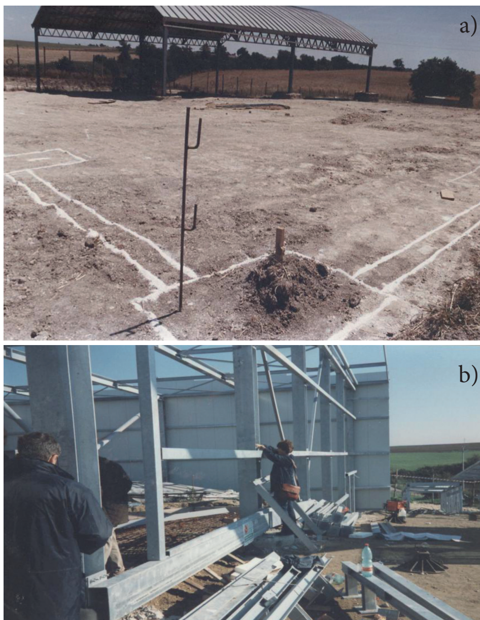
Fig. 3 - a-b) The construction of the roofing above the deposit.
