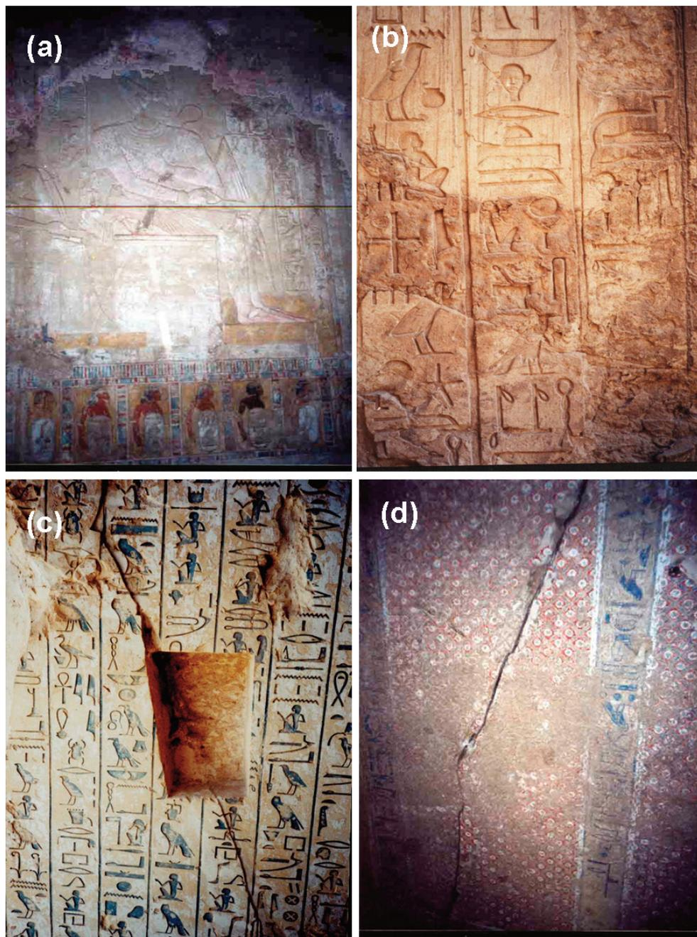
Figure 3. The decorations and deterioration aspects on the walls of tomb of Kheruef (TT192) (a): the salt layers cover the painted bass reliefs of the tomb, (b): hard crusts are observed on the surface, (c, d): macro-cracks spread on the surfaces.
