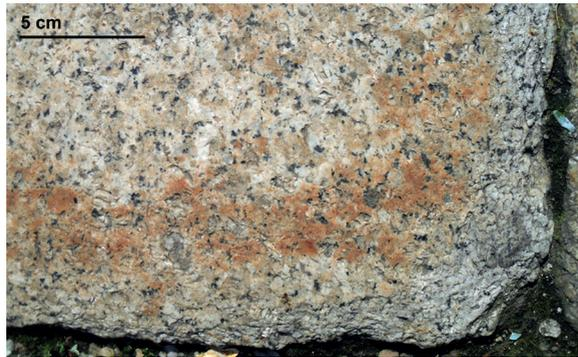
Figure 3. A paving slab of Piazza Cavalli showing rust stripes on the edges towards the sand-filled crevices.
