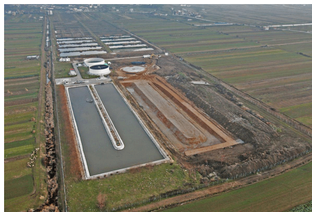
Figure 1. Wastewater Treatment Plant in Pogradec (AlbStar, 2005).
